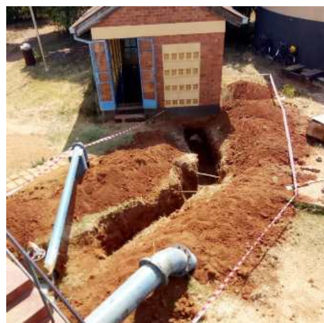
Upgrading of suction pipe from 225mm to 400mm to increase quantity of raw water getting into the treatment works for purification and distribution to residents
