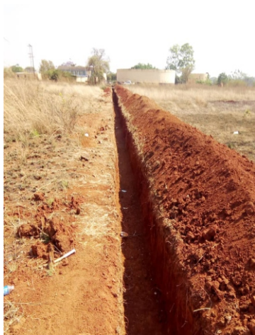
Upgrading of the main water line from current 225mm to 300mm to increase amount of treated water pumped to consumers
