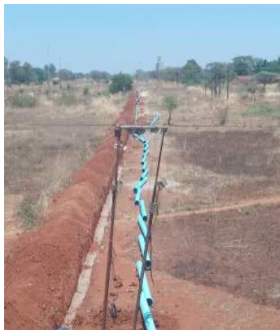
Upgrading of the main water line from current 225mm to 300mm to increase amount of treated water pumped to consumers
